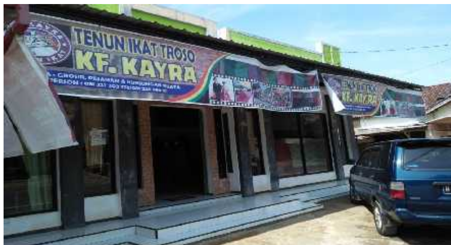
Figure 3. 32. Tenun Ikat Troso Production House, Kayra, Jepara
